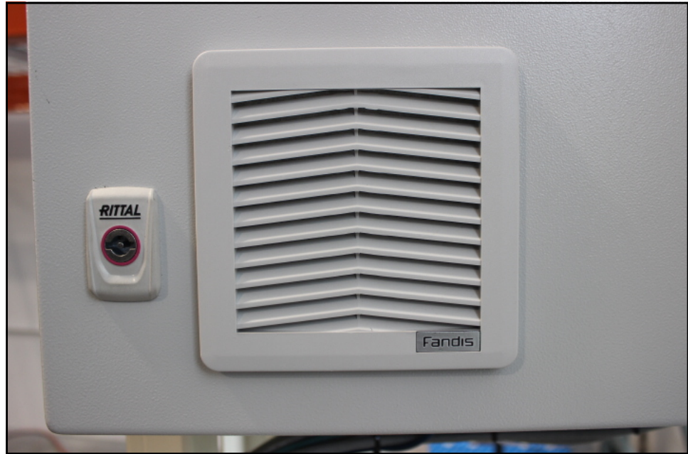
Figure 20 Control Box Front Filter
