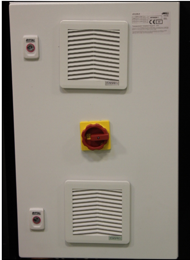
Figure 21 Control Box Filter
